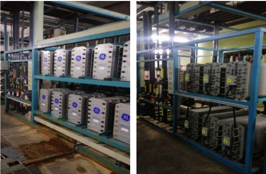
Figure: Optimized EDI system to save water
