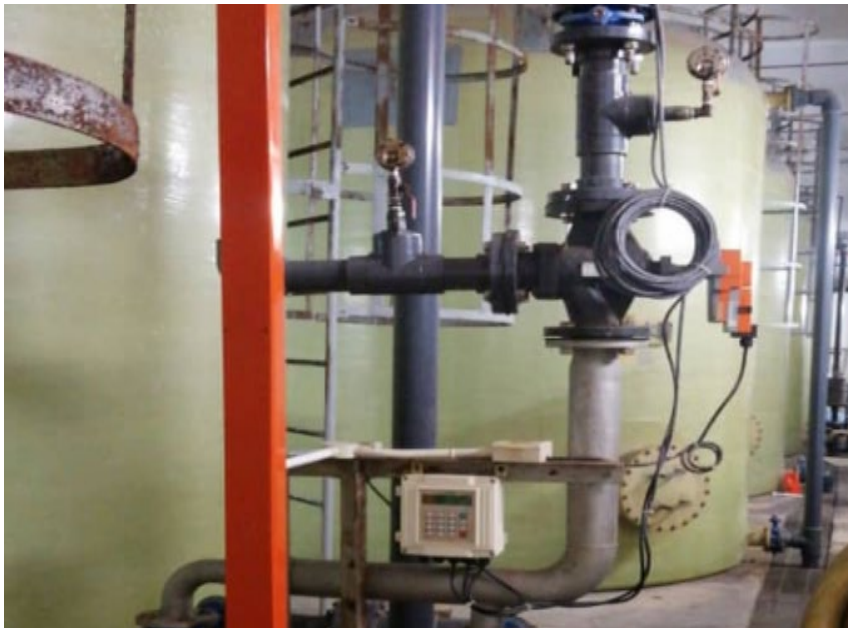
Figure: RO rejected water system
